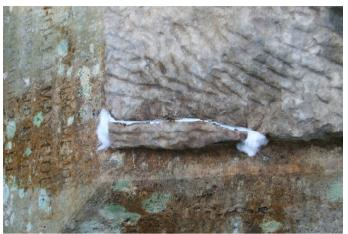
Image 6: Cracks filling after careful cleaning
